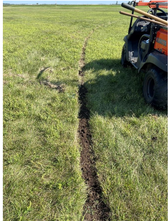
(Unknown damage in runway)
